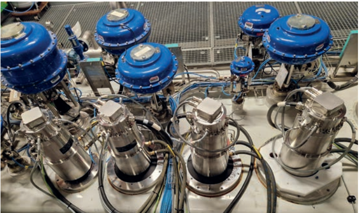
Figure 3 New cold compressor motors (metallic pillars in the front) installed in the cold compressor box
