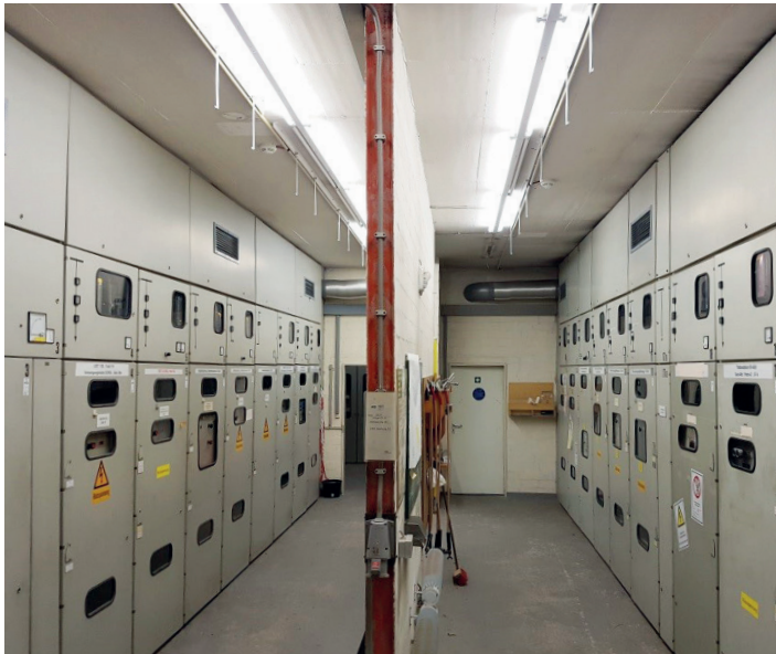
Figure 1 Left: Existing Mainstation A from 1960 with open busbar without arc fault protection and insufficient personnel safety. Right: Mainstation B, manufactured in 1975.
