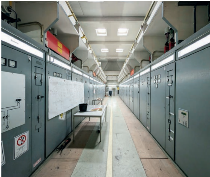
Figure 1 Left: Existing Mainstation A from 1960 with open busbar without arc fault protection and insufficient personnel safety. Right: Mainstation B, manufactured in 1975.
