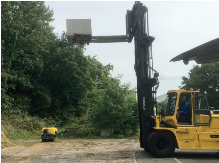
Figure 2 Dropping a 2 t shielding stone from a height of 5 m in the North area of the PETRA ring. The PETRA tunnel is only a few metres away, below the rising ridge on the left.
