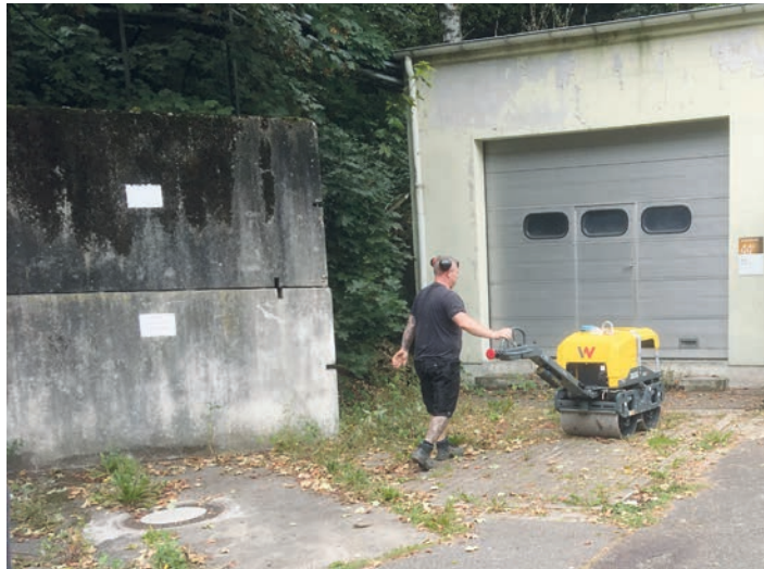
Figure 1 Ground excitation with a vibrating roller in the West area of the PETRA ring. The PETRA tunnel lies only a few metres to the left. The shielding stones in front of the material side entrance are visible on the left.
