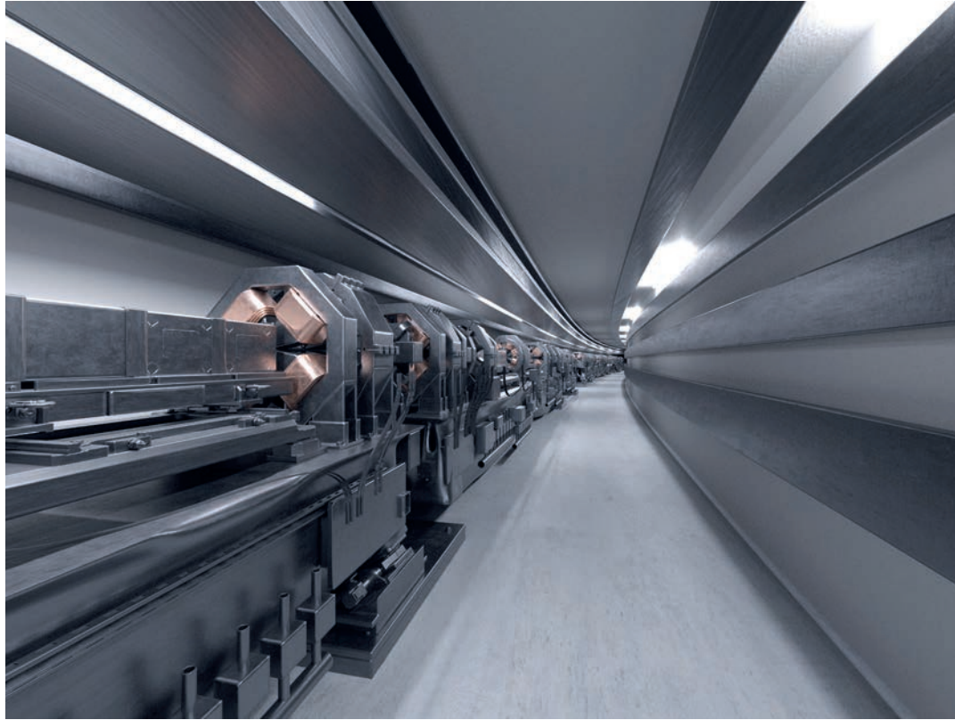
Figure 3 Visualisation of the view into the PETRA IV tunnel with assembled girders
