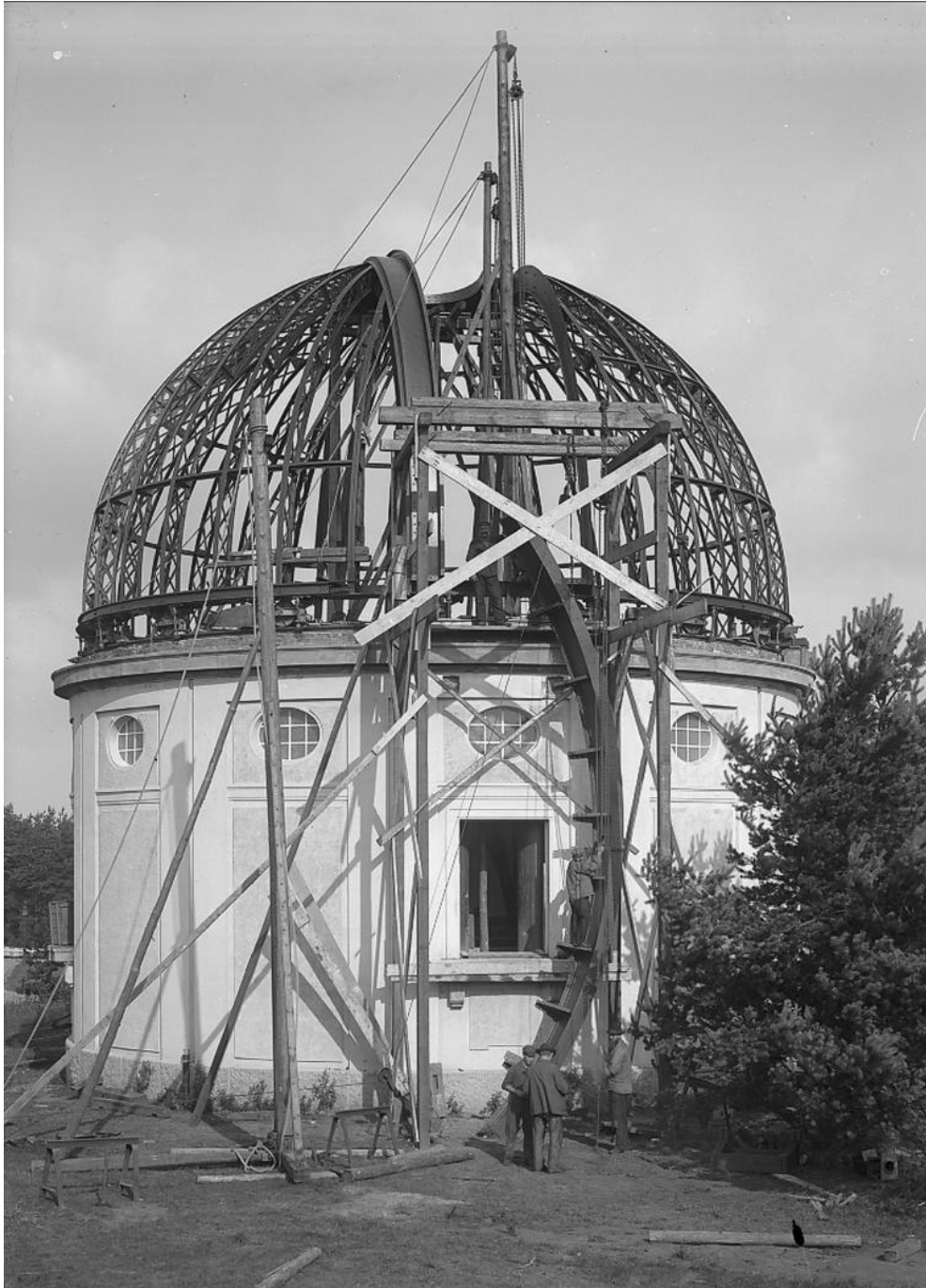
Figure 2: The Great Refractor dome under construction in 1910. Credit: Photographic Archive of the Hamburg Observatory
