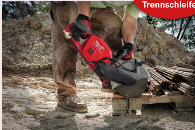
(Foto: Milwaukee Electric Tool Corporation)
