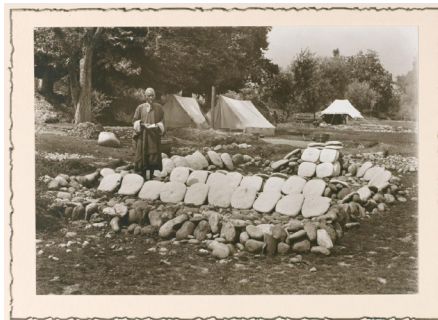
Fig. 4. Pulp cakes bleaching in the field.
