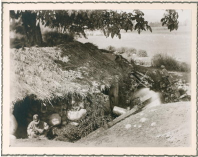
Fig. 2. Pulp beating under the wooden stamper, the water wheel.
