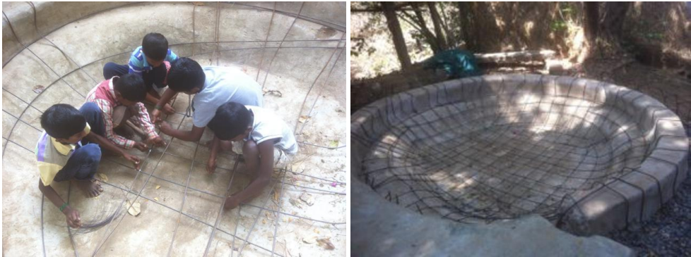
Figures 5 & 6: Building mesh structure
