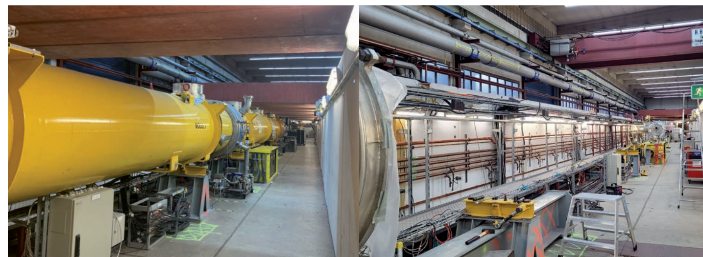
Figure 2 Shutdown work in the FLASH injector section. Two accelerator modules (left) are removed (right) to be replaced by upgraded modules.
