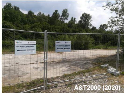
Figure 12: Area of the installation of the mAD plant and current biomass platform
