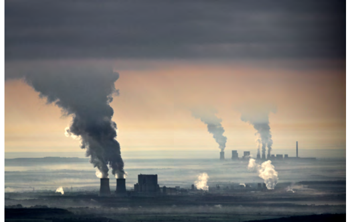
Aerial view of brown coal (lignite) power plants in Germany
