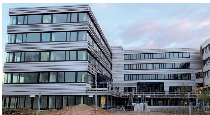
Figure 1 Construction of the CXNS building is almost completed.
