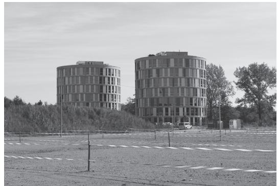
Abb. 23: Nordport Towers in Garstedt
