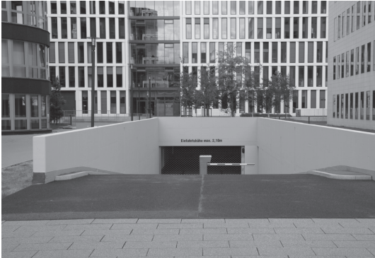
Abb. 10: Airport City Parkgaragen
