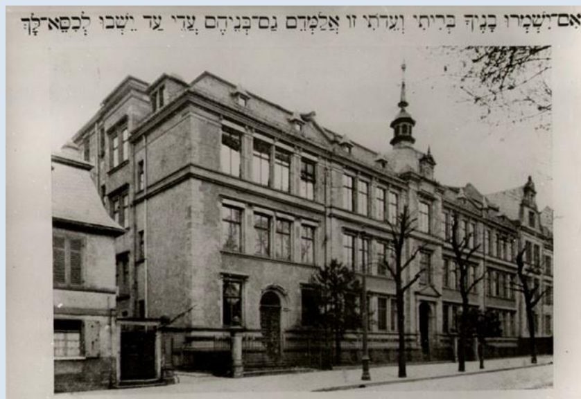
The Real-School building, Frankfurt on the Main, Germany, photo taken on 1928
