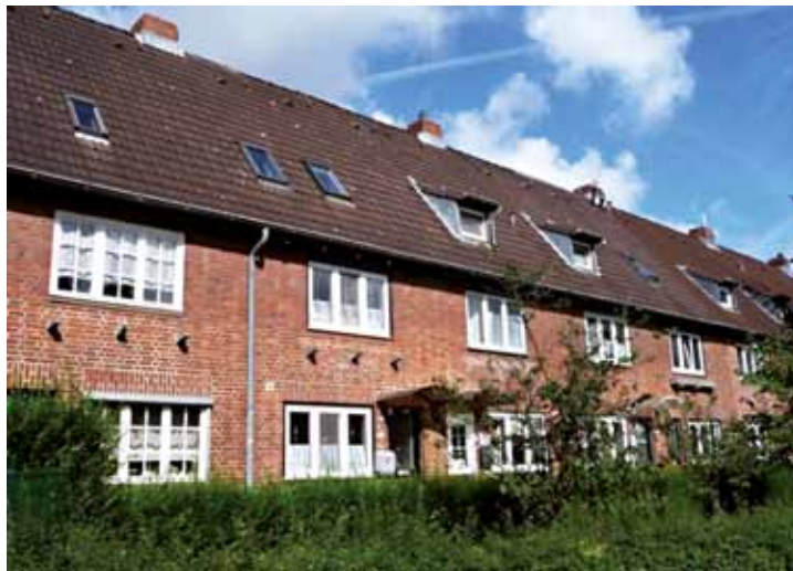
Figure 1: Row house, 'Kiel Elmschenhagen-Nord'
