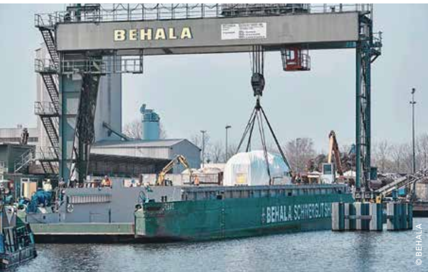
BEHALA also loads Siemens gas turbines for export through Hamburg by crane at its Berlin plant
