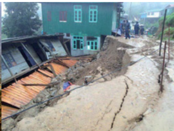
Hakha after the floods of 2015
