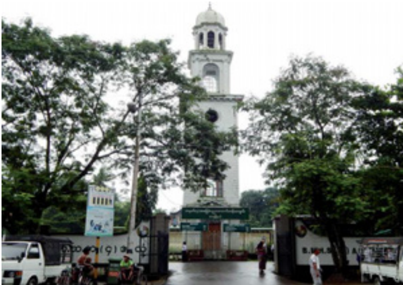
The former Cushing High School, now Basic Education High School No 4 Ahlone. The building is listed on the Yangon Heritage List. (For another picture of the school see biography 4.)
