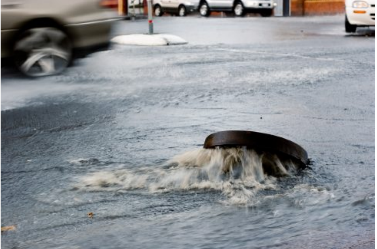
Fig.1. Overflowing sewage system following an extreme precipitation event. © iStock/Dizzy
