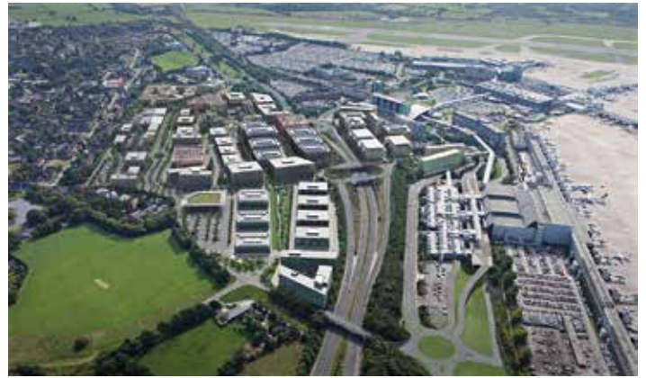
Airport-City Manchester, England
