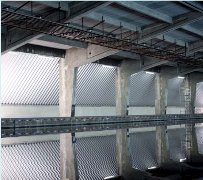
Fig. 1: Building extension ready for the installation of the Side Wave Generator
