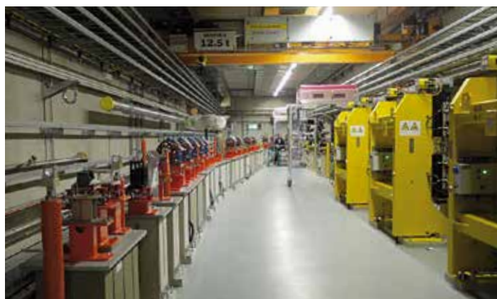
Construction of the beamline (left) connecting the FLASHForward experiment to the FLASH accelerator
