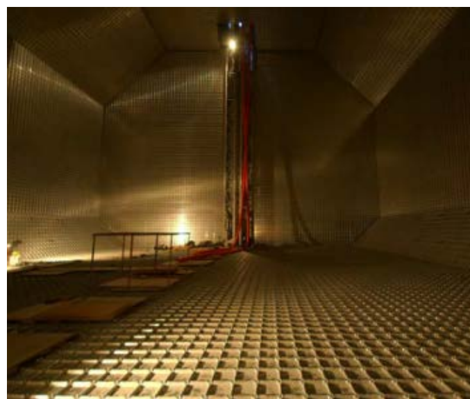
State-of-the-art membrane tanks make the best use of the available space and are safe and highly resilient, thanks to the creased wall structure.
