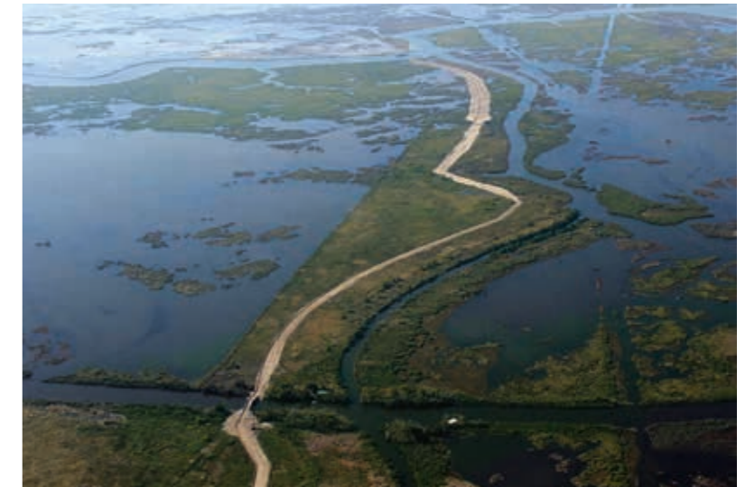
4.21 > Since 2013, sand from the Mississippi River at New Orleans has been pumped through a pipe for a distance of over 20 kilometres into the delta. Sand banks are created on which many square kilometres of salt marsh can develop. These, in turn, act as natural coastal protection.
