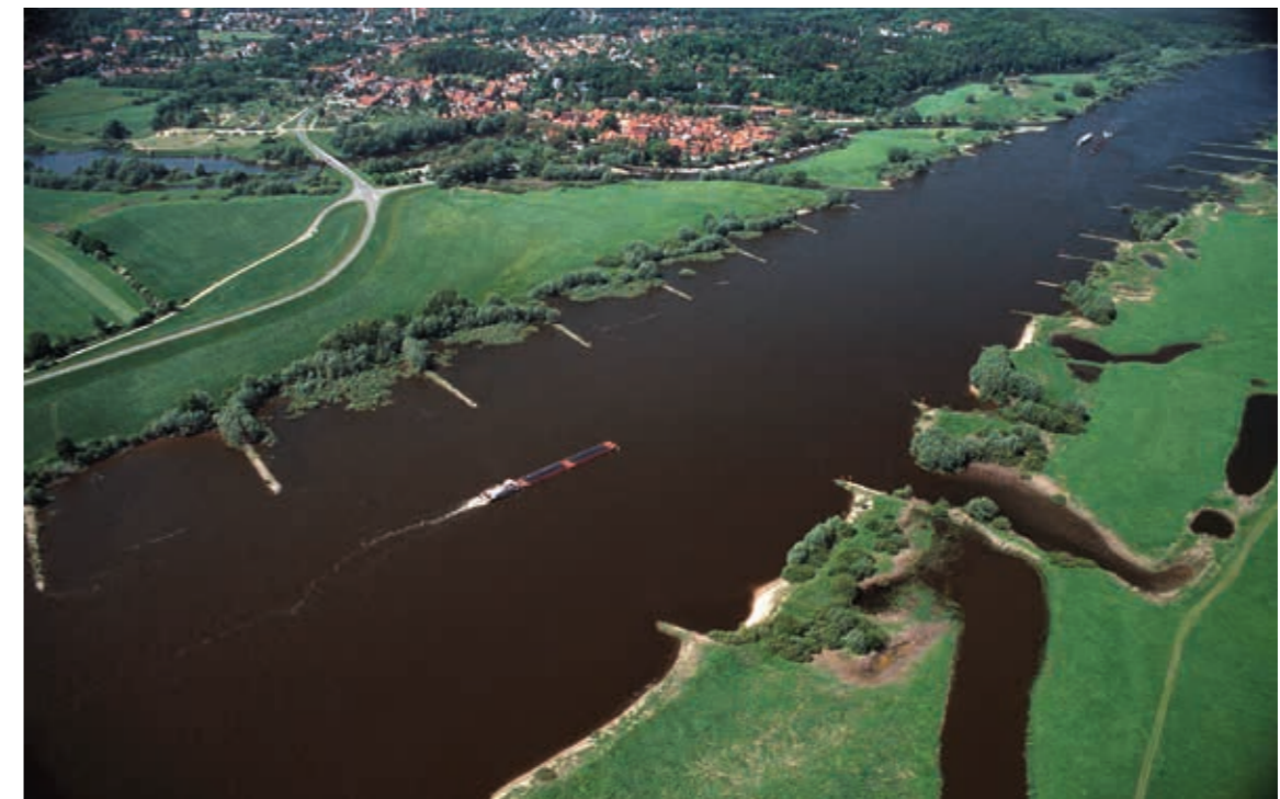
4.3 > Responsibility for the maintenance and safety of federal waterways like the river Elbe, pictured here, rests with the Federal Ministry of Transport and Digital Infrastructure, whereas the dikes protecting the hinterland are cared for by dike associations.
