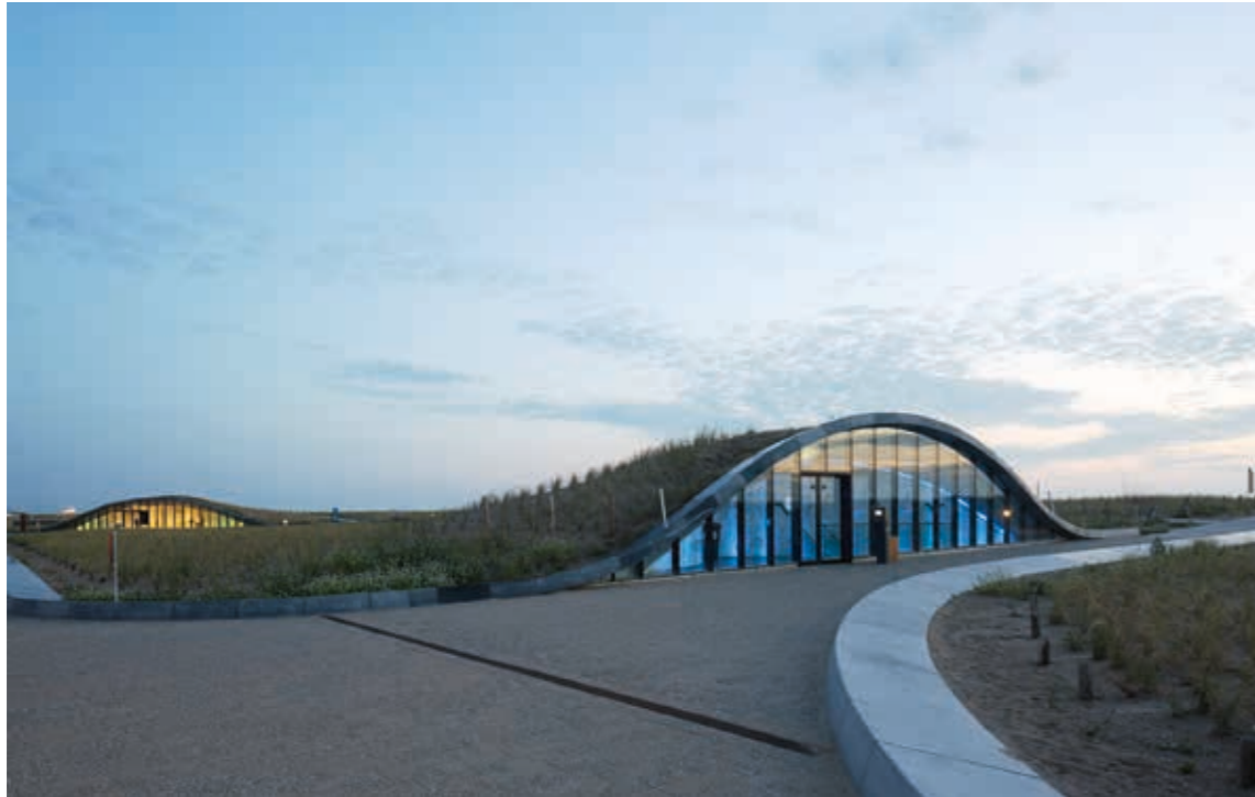
4.27 > In the Dutch resort town of Katwijk aan Zee, a parking garage was built parallel to the shore road and then covered with sand to create a high artificial dune.
