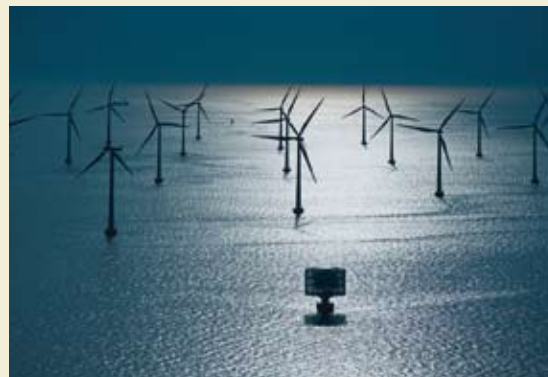
7.12 e > Offshore wind turbines produce electricity in many places around the world. One of the largest offshore wind farms, consisting of 48 turbines, is located in the Baltic Sea between Denmark and Sweden. A transformer station has been constructed here to feed power into the Swedish grid.
