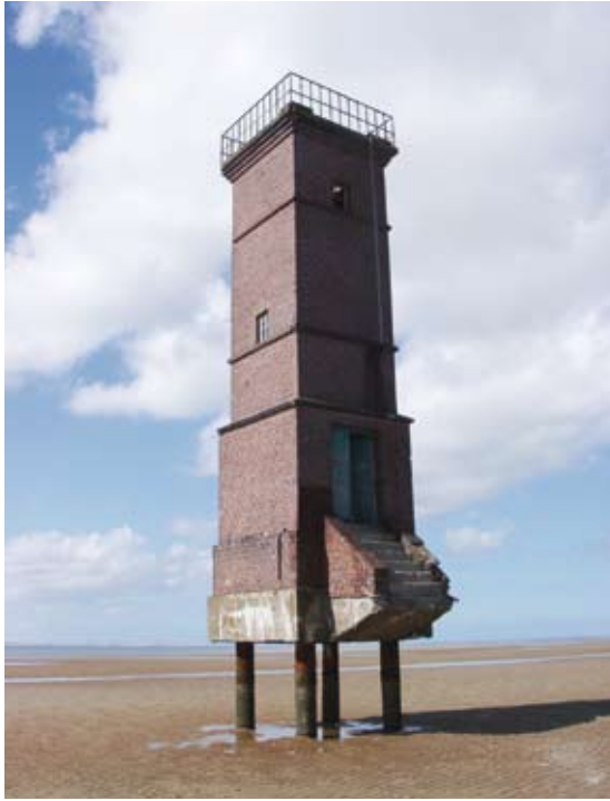
3.7 > The old lighthouse on the East Frisian island of Memmert once stood in the dunes, but was washed out by erosion over the course of decades.
