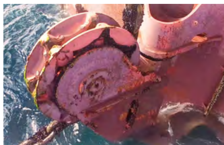
Wind conditions and the flying distances make offshore drone surveys a particular challenge for drone surveyors.
