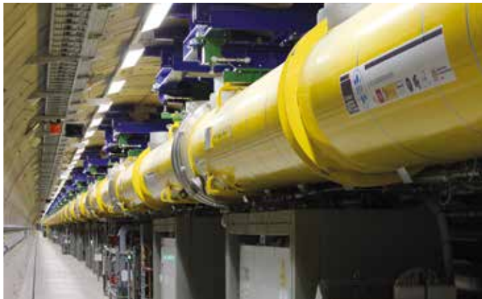
Figure 1 European XFEL main accelerator ready for cool-down at the beginning of December 2016
