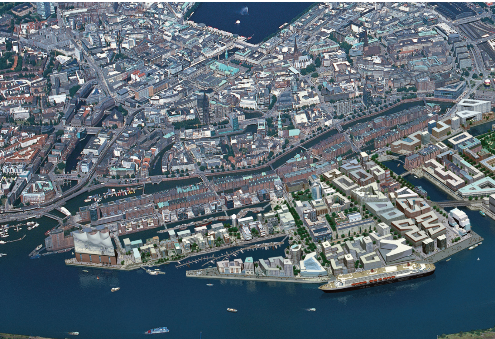
Western and central HafenCity
