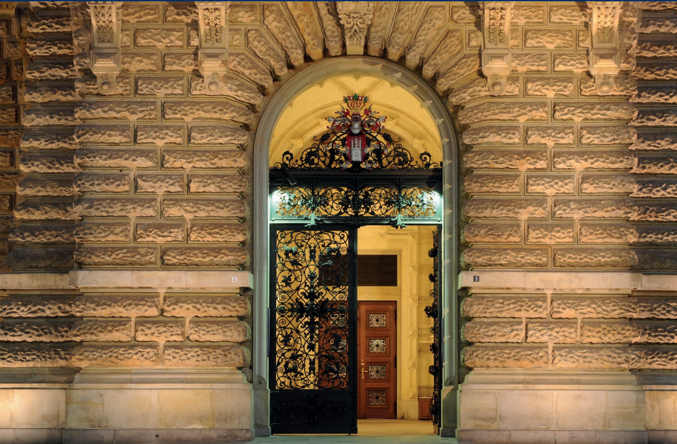
Cast iron gate – Entrance to the Rathaus
