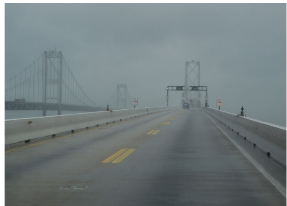
Chesapeake Bay Bridge closed in anticipation of Hurricane Isabel in 2003. Credit: FEMA.
