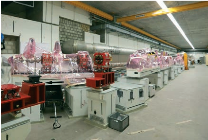
Figure 2 View into the injector tunnel (November 2014)
