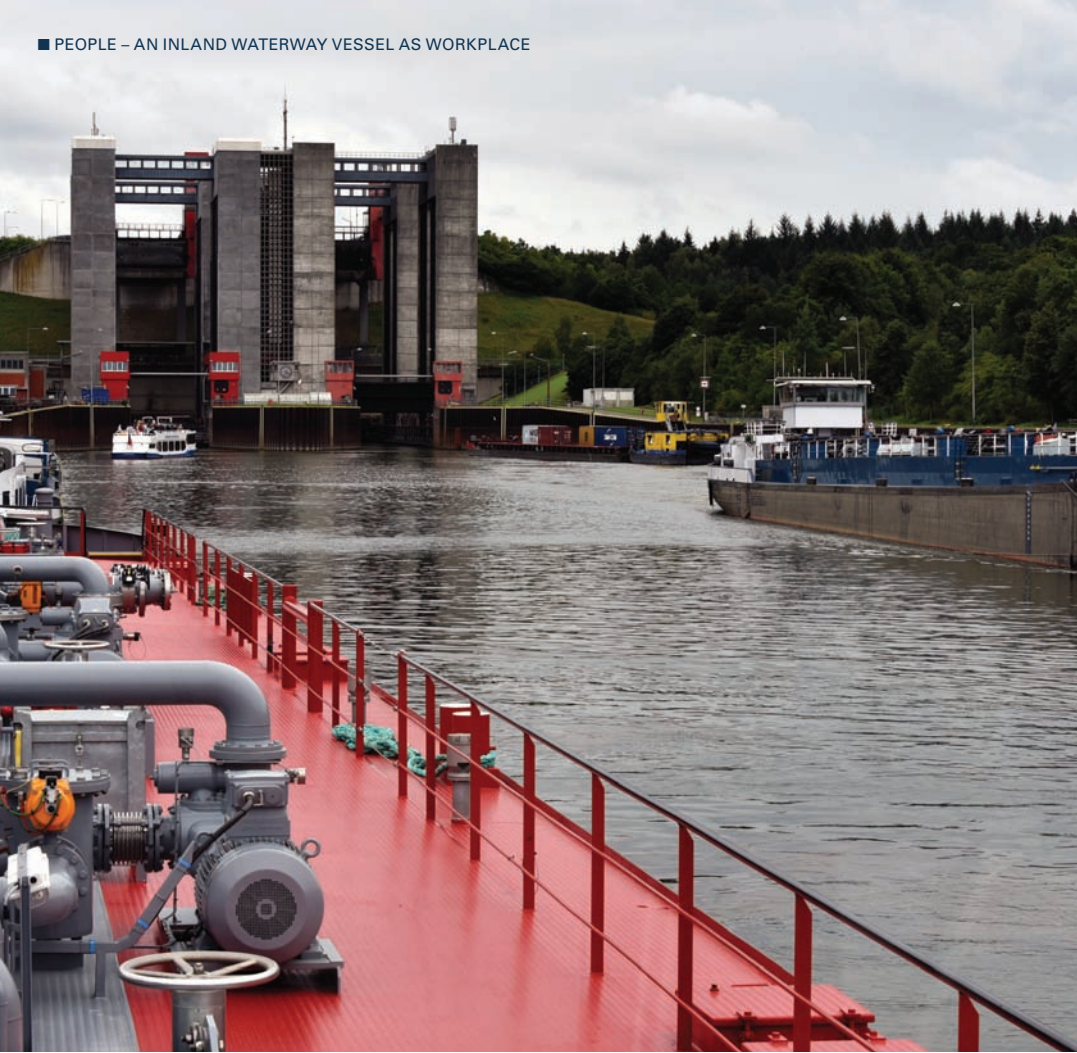
Entering a trough at Scharnebeck lifts requires the utmost concentration. On each side a gap of just 27 centimetres remains between the ship's hull and the lock wall
