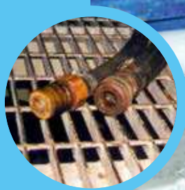
Quick-disconnect, flexible hose connections for the cooling water system.
