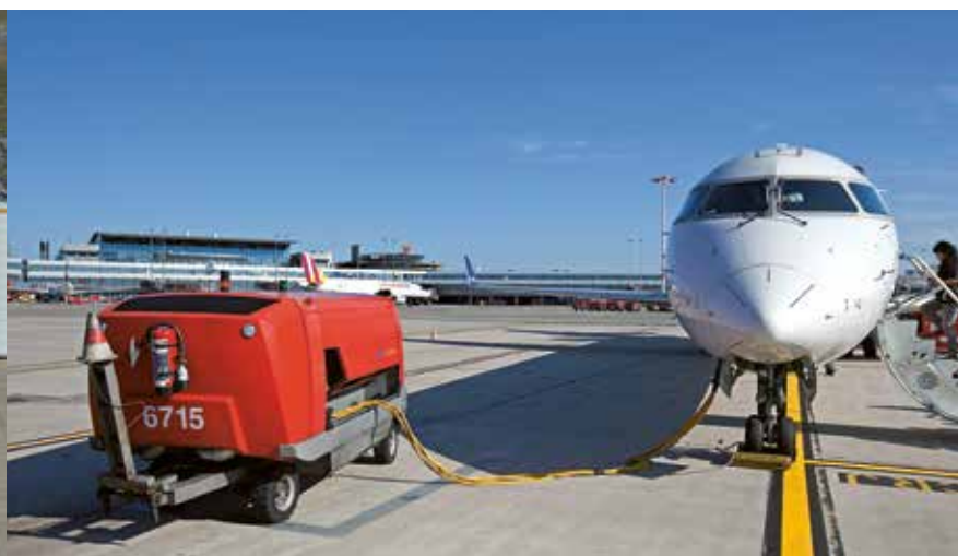
Mobile generators supply aircraft at remote parking positions with electricity, so that the APUs are not needed here, either
