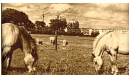
Baustelle Osdorfer Born
