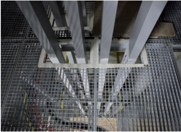
Figure 3 Waveguides in the European XFEL injector shaft
