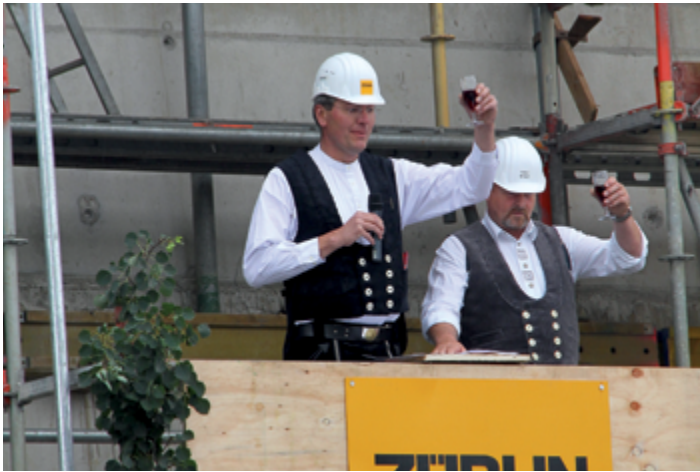
Topping-out ceremony for the FLASH II experimental hall
