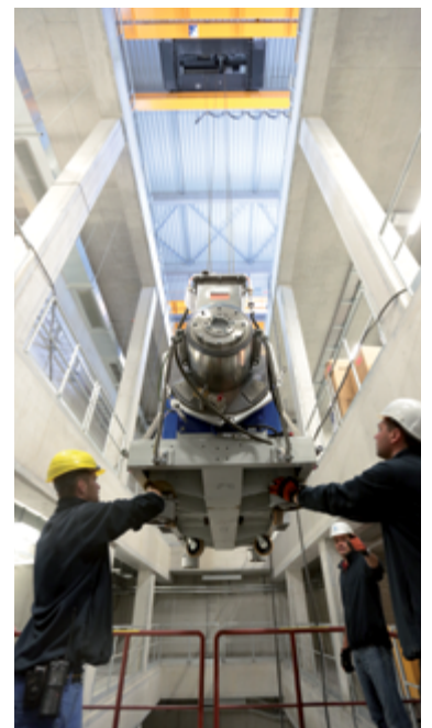
Installation of klystrons in the European XFEL injector building in August 2013
