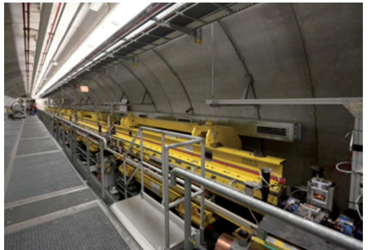
Tunnel of the FLASH free-electron laser
