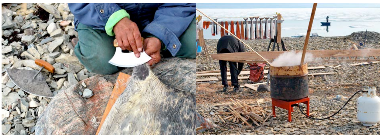
Figure 26. Left: Mary Avalak uses an ulu knife to shave the hair from a sealskin in preparation for creating the kayak cover. Right: A propane tank is used to heat water to steam kayak ribs for bending.
