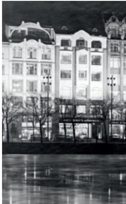
Above: The Alsterdamm in the mid-1930's. The TROPAG offices were located on the two upper floors of Number 7 (left).
