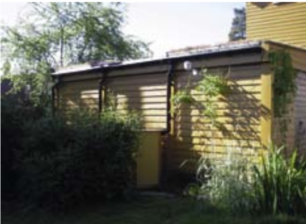
Green vegetative roofs
