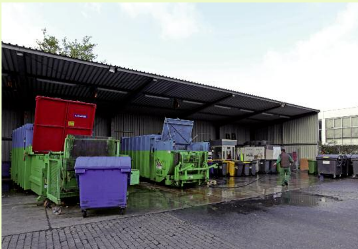
Waste collection area
