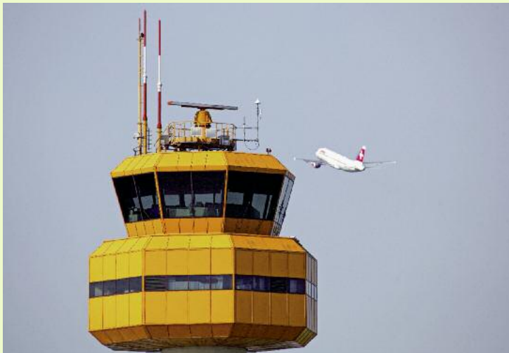
German Air Traffic Services (DFS) airspace monitoring control tower
