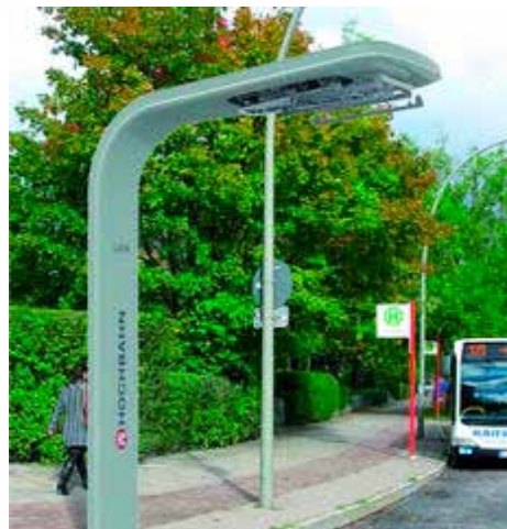
E-Bus Ladestation. Quelle: HVV
