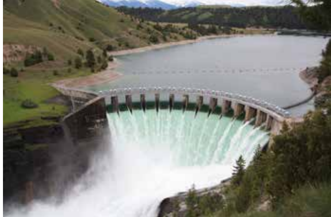
Kerr Dam with all gates flowing
