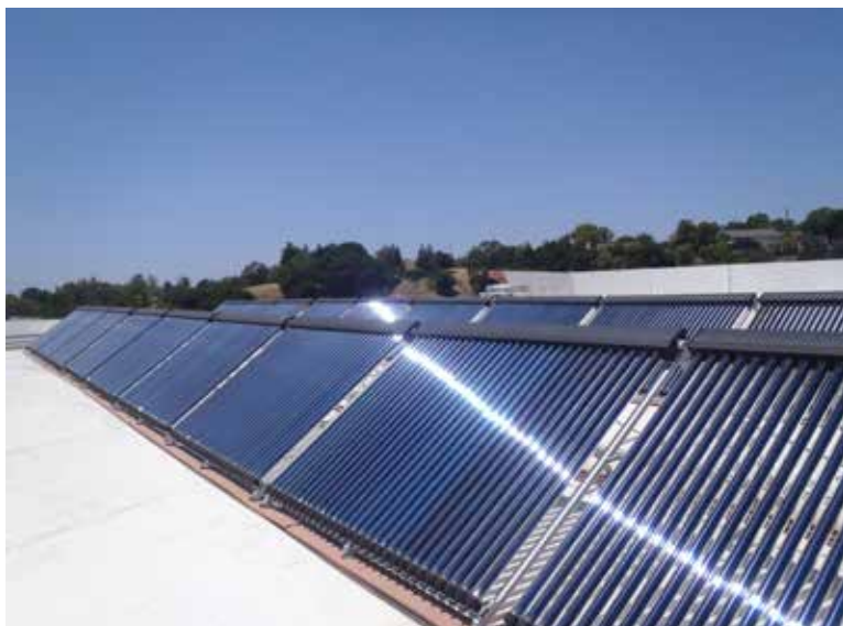
Solar thermal collectors at the Chumash Casino
