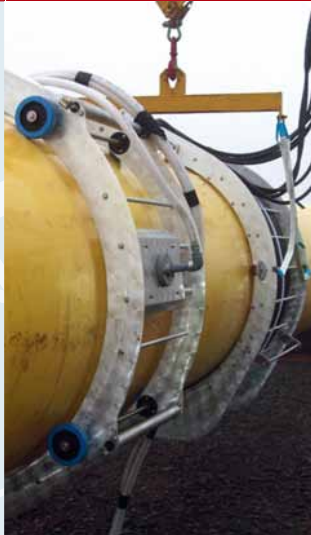
FIGURE 1. Induction heating coil and powder spray units.
