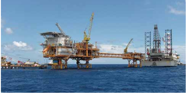
PRODUCTION. The PUQC topside (Production Utilities Quarters Compression-Platform) in the Rong Doi-Field about 320 kilometres offshore Vietnam.
