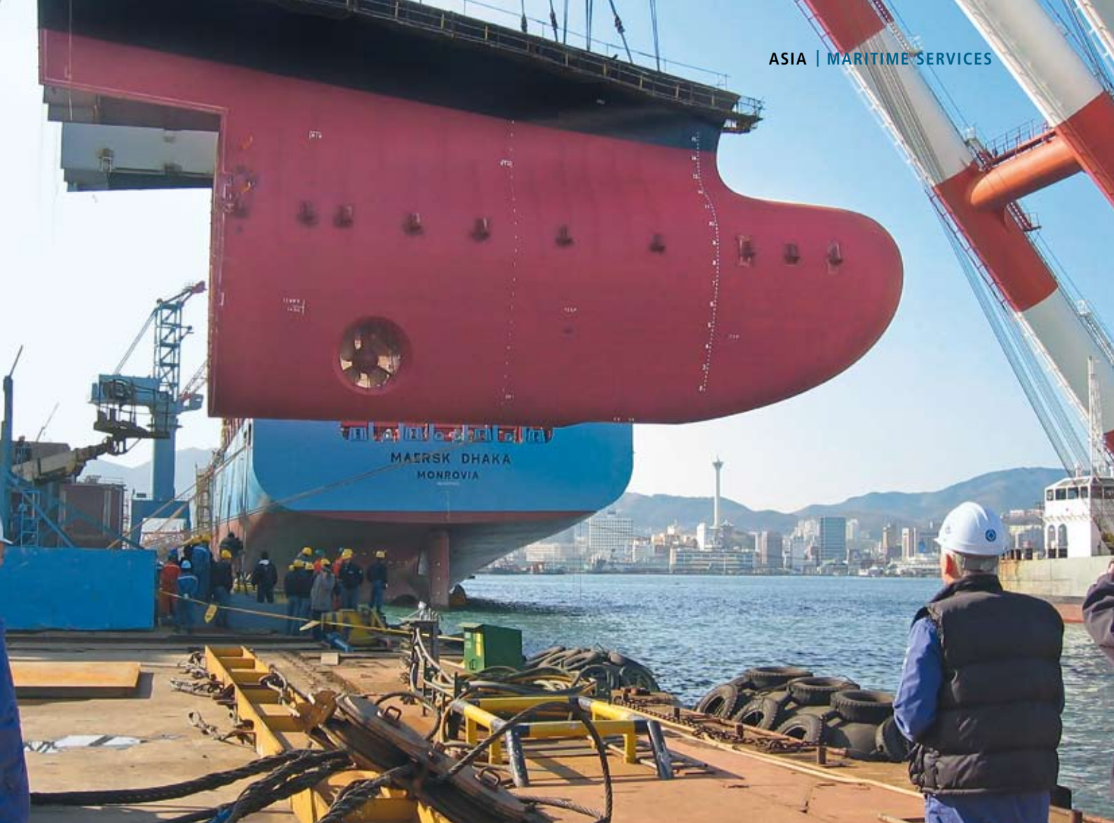
SHIPBUILDING KIT. At Hanjin Shipyards, a ship is being assembled applying the “DAM” system. The main hull and the bow section are completed as separate units, then welded together, allowing the shipyard to build ships larger than the dock.
