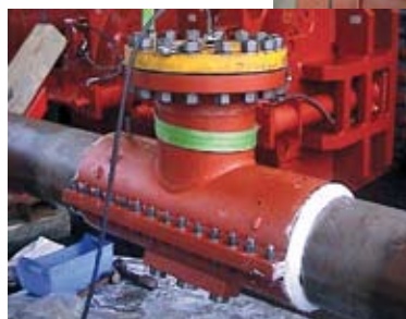
APPLICATION. The alternative solution for the installation of welded T connections in live gas pipelines is safe and versatile.
