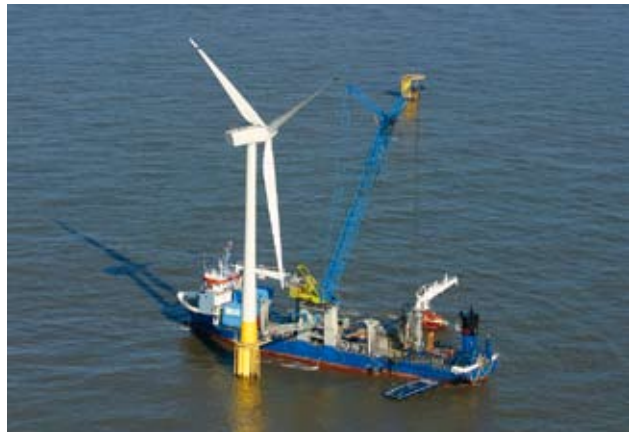
SOPHISTICATED. Installation of a rotor blade at the Scroby Sands wind farm located in the North Sea, 2.5 km off the coast of eastern England.
