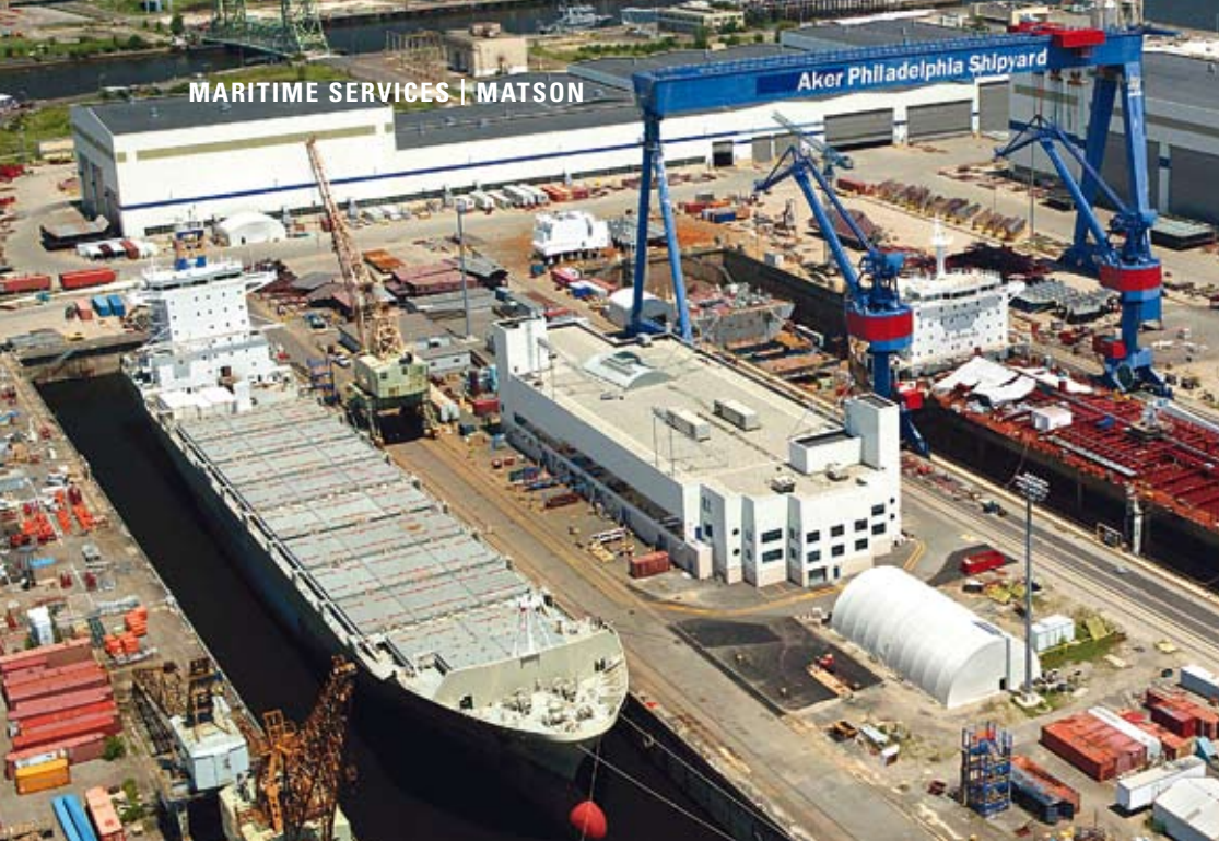
SHIPBUILDING. The GL-certified Maunalei at Aker Philadelphia Shipyard.
