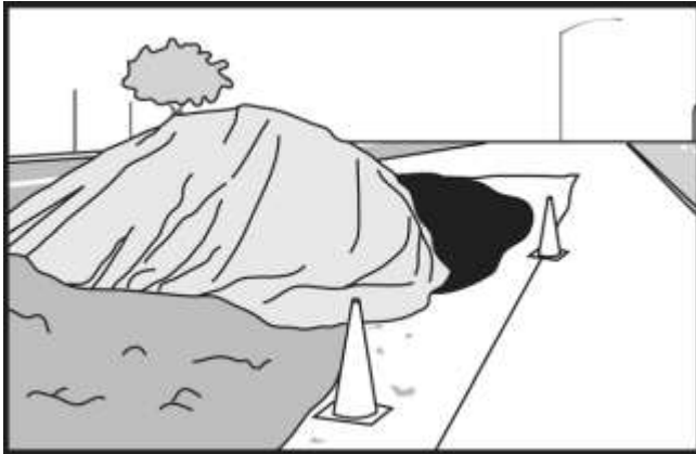
Figure 17: Impermeable Membrane Under and Over Excavated Fill
