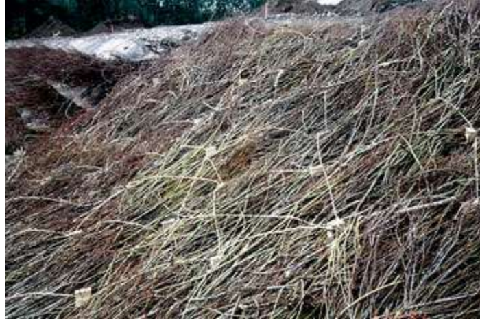
Figure 26: Brush Mat Re-Vegetation Technique
