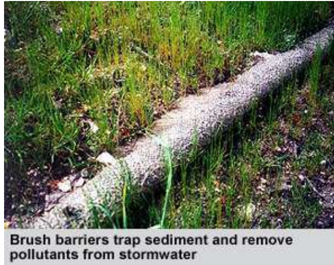
Figure 23: Brush Barrier Used for Sediment Control
