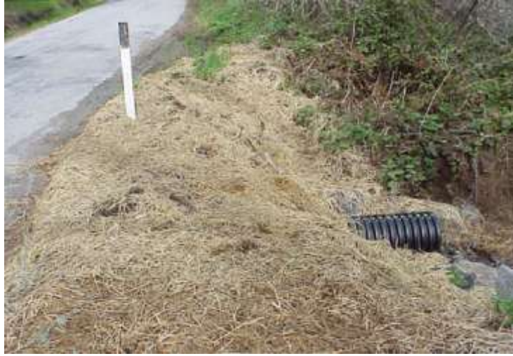
Figure 19: Using Straw Mats to Protect Exposed Areas Prior to Re-vegetation
