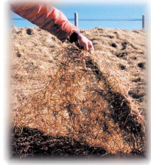
Figure 19: Using Straw Mats to Protect Exposed Areas Prior to Re-vegetation
