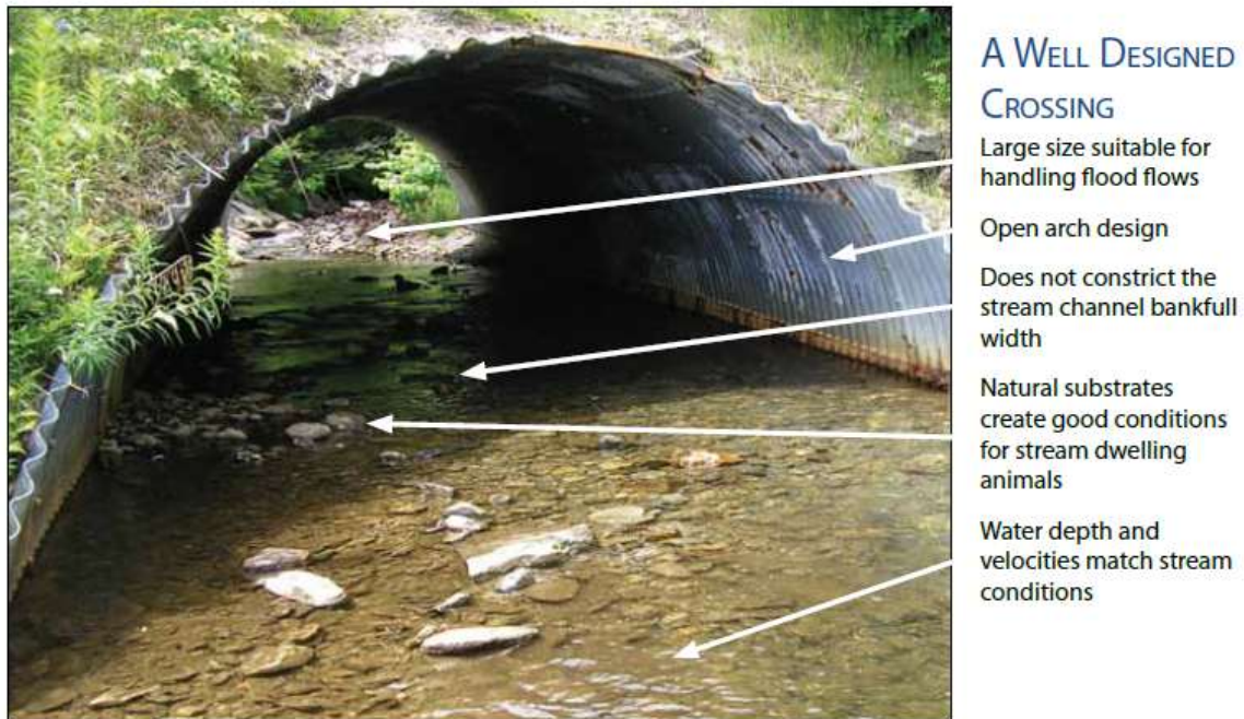
Figure 13: Characteristics of a Well-Designed Creek Crossing
