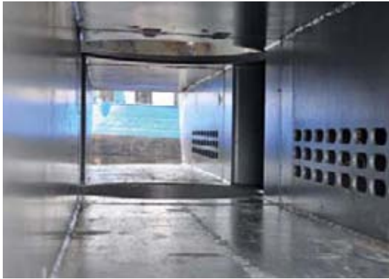
TUNNEL. Bow thrusters improve the vessels' manoeuvrability.
