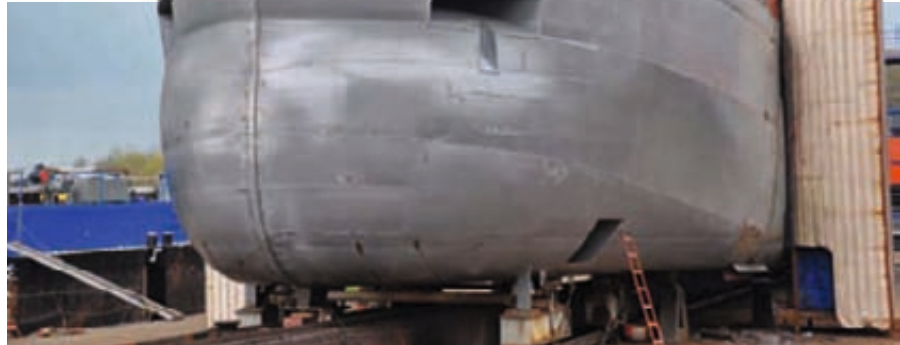
STEELWORK. The enhanced hull design reduces the weight by 20 per cent.
