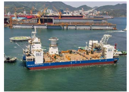
“VICTORIA MATHIAS”. Powerful cranes, but still no forebody.
