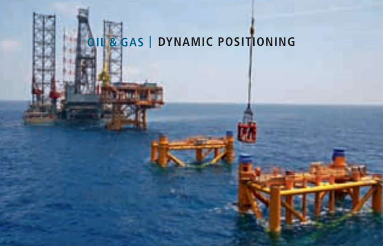
FLOAT-OVER. Phases of an operation: The installation of a topside onto a pre-installed jacket by means of an installation barge.
