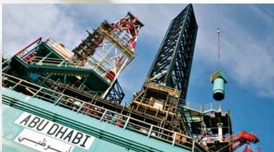
Conversion. GL supervises the modernization of drilling rigs.
