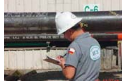
PIPELINES. An MCS expert performing quality tests on pipes.
